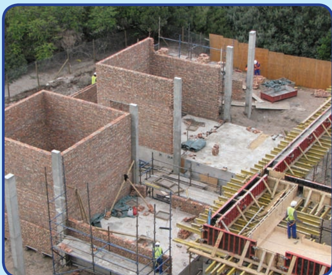
Photo of early stages of building site shows the large concrete block which reduces vibrations in the rooms
