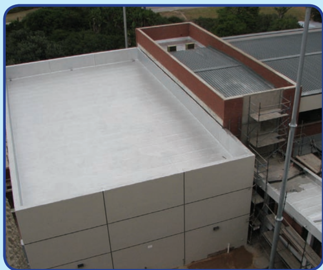
HRTEM rooms are housed within this section with special features
